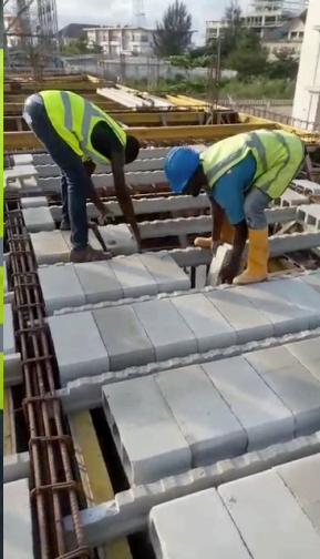
Placing Hollow-Pots
