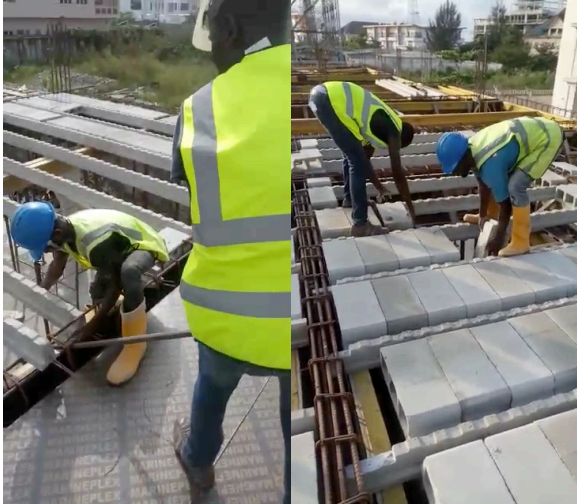
Positioning Ribs
