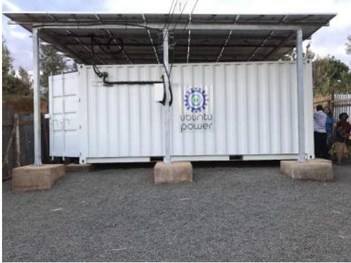
A 20kW mini-grid serving 110 households in Mutaroni Village in Tharaka Nithi County in Kenya.
