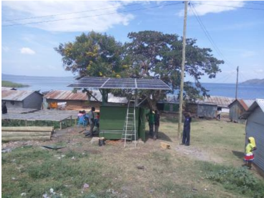
A mini-grid serving 27 households in Ragwe in Homa Bay County on the shores of Lake Victoria.
